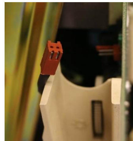
Figure 64 VT220 double câble retiré © HE-Arc, N. Nydegger, 2019
